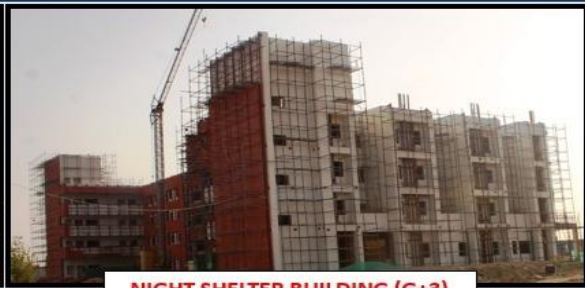
NIGHT SHELTER BUILDING (G+3)
