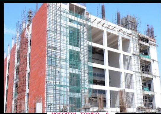
HOSPITAL TOWER - 6, OPD Block (B+G+4)
