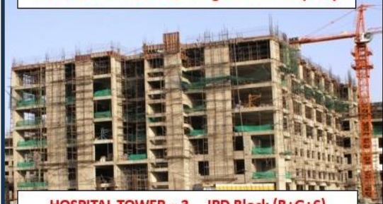
HOSPITAL TOWER - 3, IPD Block (B+G+6)
