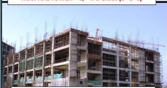
HOSPITAL TOWER - 5, IPD Block (B+G+6)
