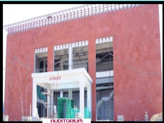
AUDITORIUM BUILDING (G+1)
