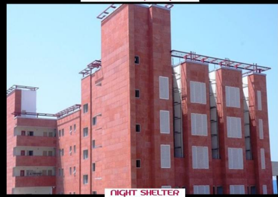
NIGHT SHELTER BUILDING (G+3)
