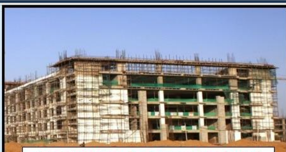
HOSPITAL TOWER - 2, Emergency Block (B+G+4)
