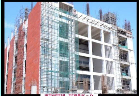
HOSPITAL TOWER - 6, OPD Block (B+G+4)
