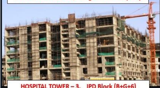
HOSPITAL TOWER - 3, IPD Block (B+G+6)
