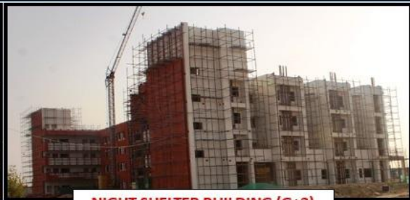
NIGHT SHELTER BUILDING (G+3)
