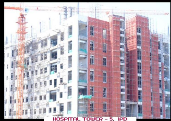
HOSPITAL TOWER - 5, IPD Block (B+G+6)
