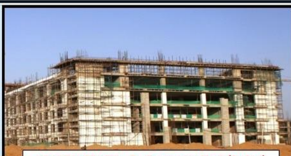
HOSPITAL TOWER - 2, Emergency Block (B+G+4)
