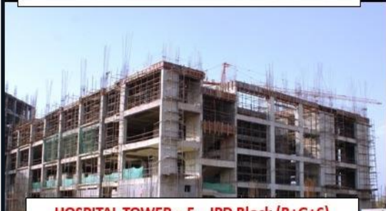
HOSPITAL TOWER - 5, IPD Block (B+G+6)
