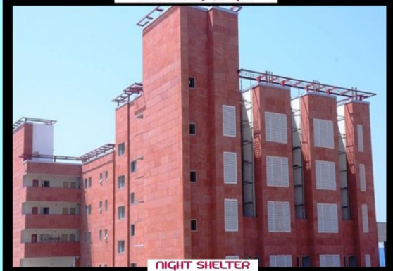
NIGHT SHELTER BUILDING (G+3)
