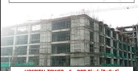
HOSPITAL TOWER - 6, OPD Block (B+G+4)
