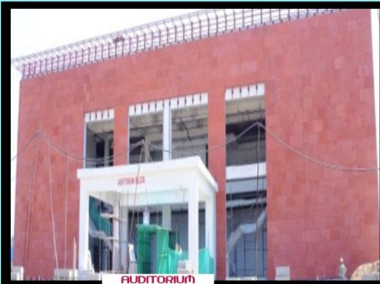
AUDITORIUM BUILDING (G+1)
